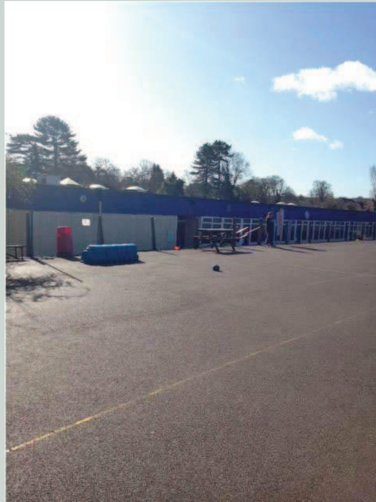
Fig 1 : site of extension showing existing rear elevation of school and change in site level
