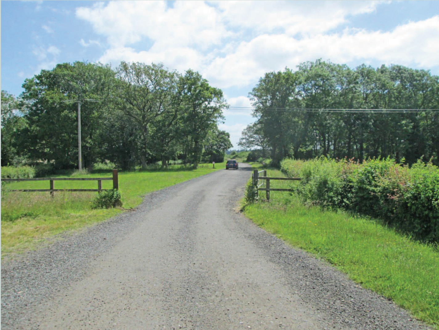
Fig 1 : Start of Existing Agricultural Track off Henfold Lane
