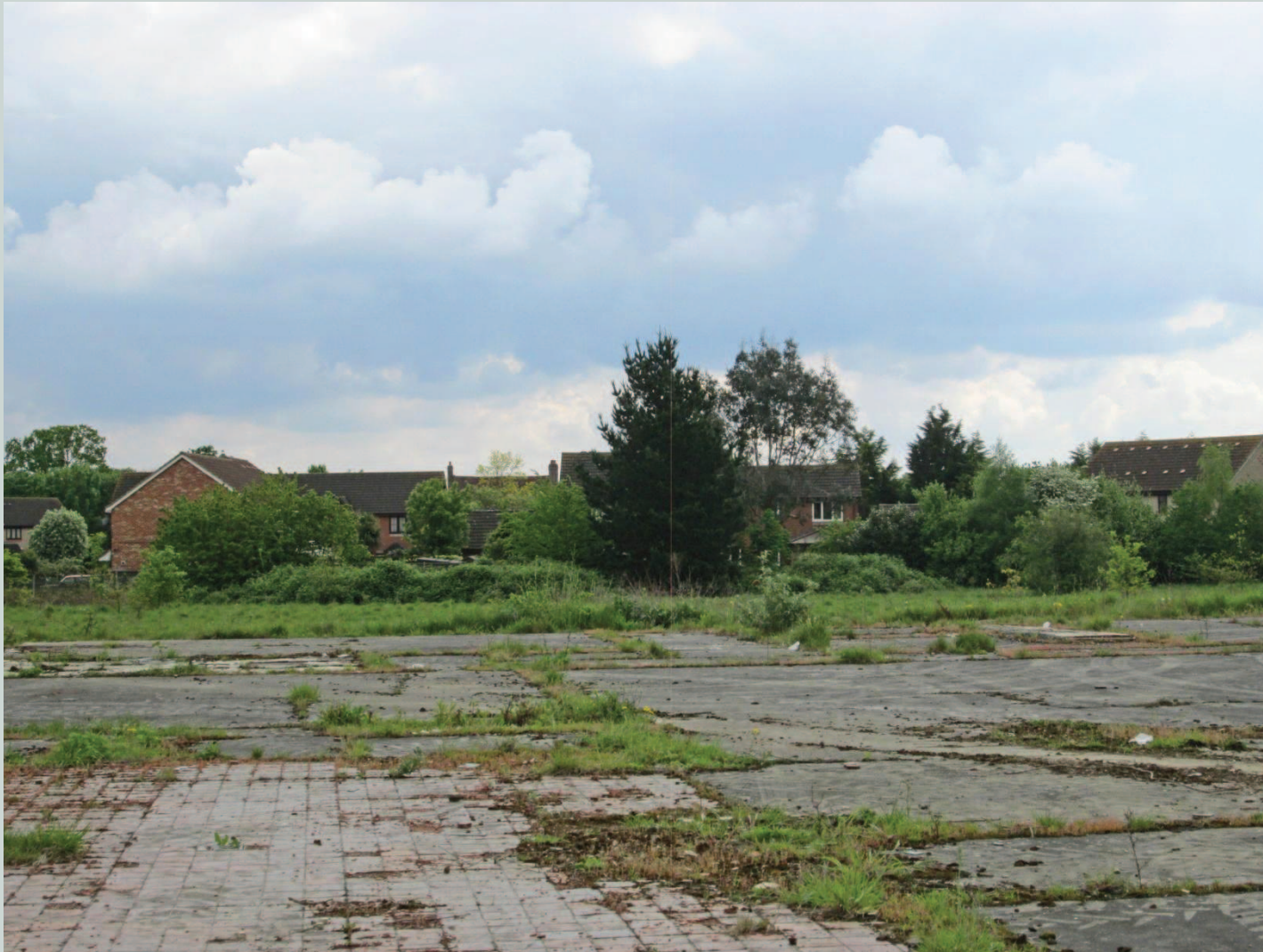
Fig 11 : Looking south from plateau towards houses in Weldon Drive
