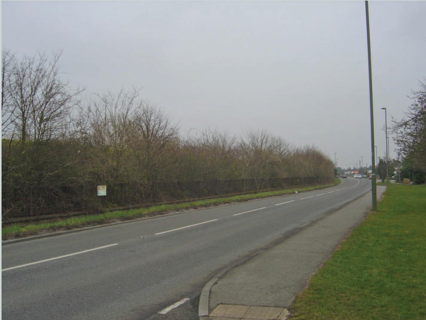
Fig 4 : View looking east along Hurst Road from near western entrance to site
